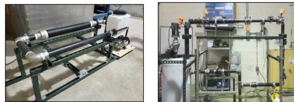
Pipe Loops at FIU – Bench Scale and Engineering Scale
