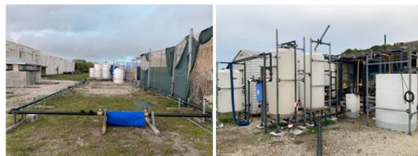
Pipeline constructed for flushing experiments at FIU
